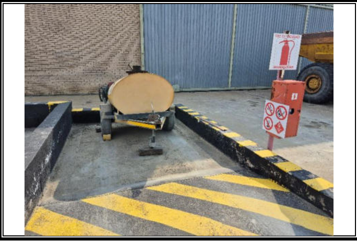
Bunds to be sealed and the integrity tested
