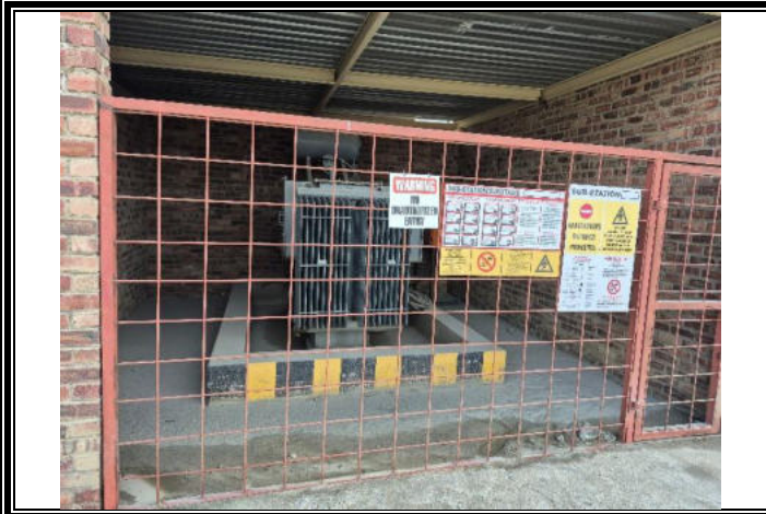
Bund wall in place
