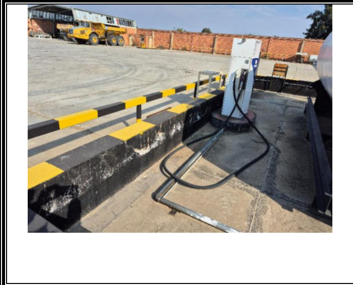
Bunds to be sealed and the integrity tested
