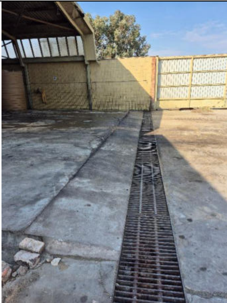
Drain of wash bay cleaned
