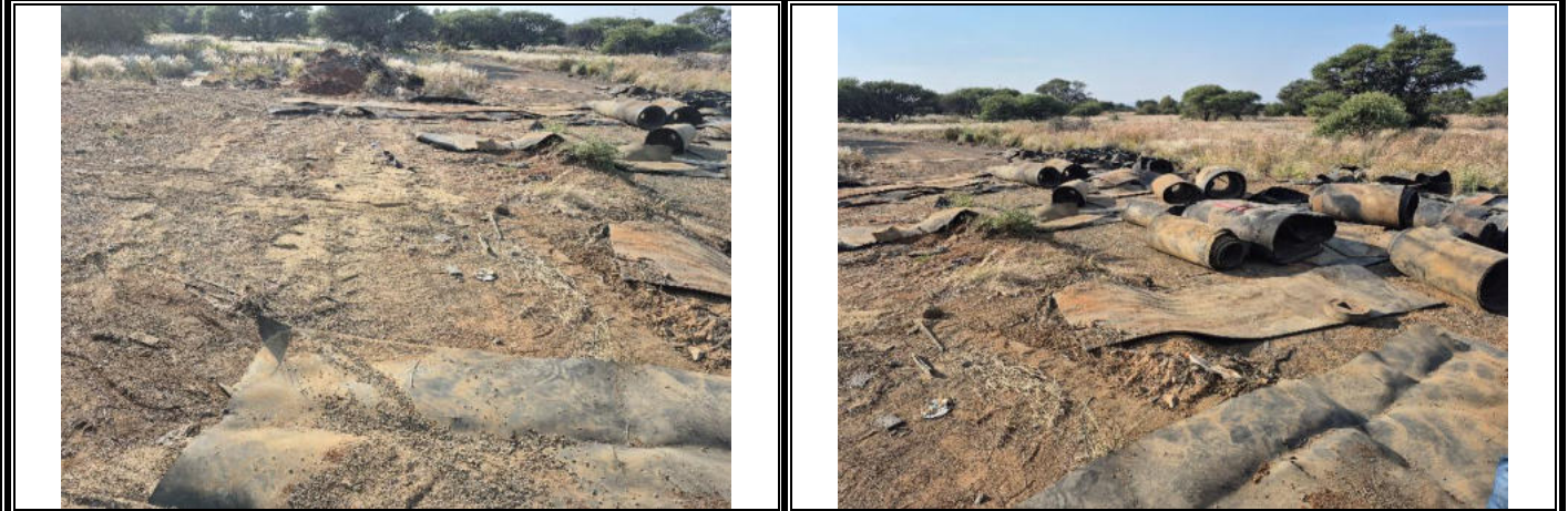
Conveyor belts being removed from site
