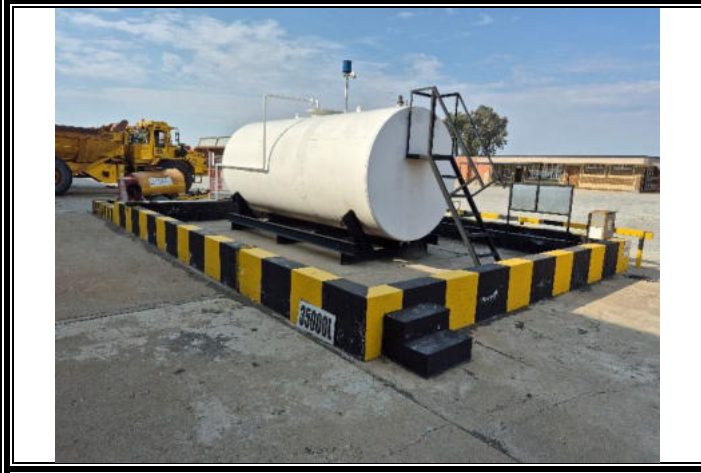
Bunds to be sealed and the integrity tested
